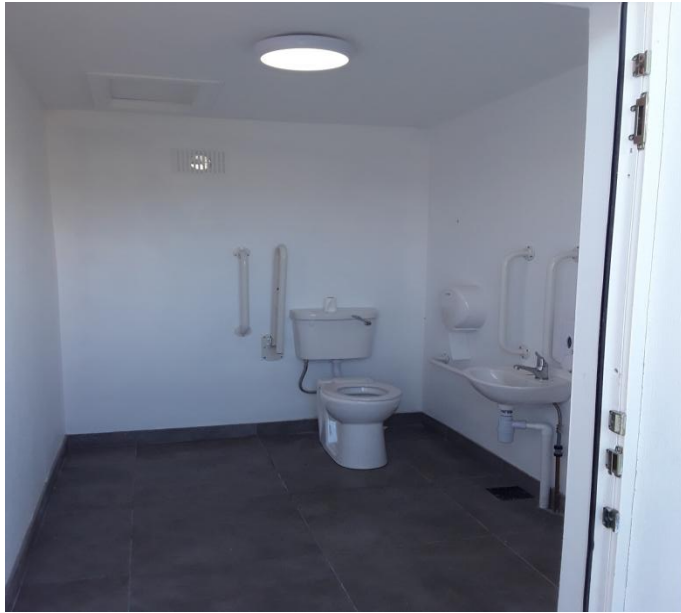
1. The fully accessible toilet unit.
